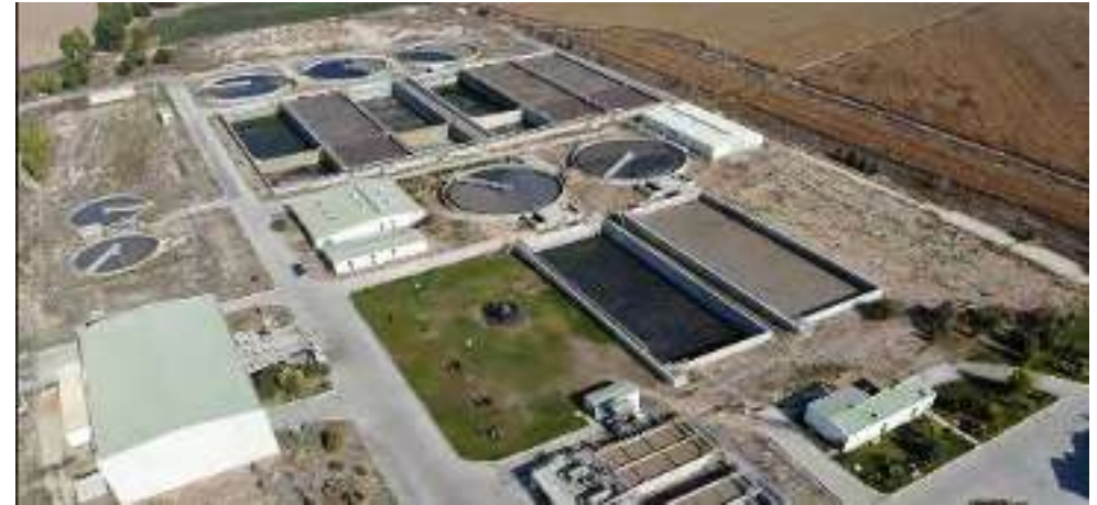
EOSB Waste Water Treatment Plants
